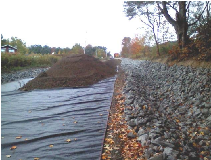
Example of geotextile fabric being used to protect ditch and roadbed from contamination.
