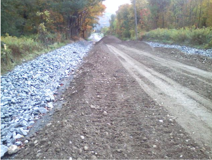
Example of gravel replacement being tied in with armored ditches. Geo textile fabric will be used under the stone in the ditches and under the gravel in the roadway to further mitigate possible contaminants moving "up" through the materials resulting in erosion.
